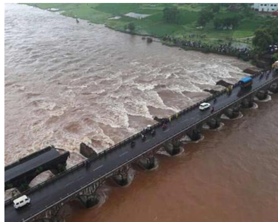
Fig. 1. Collapsed Mahad bridge
