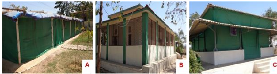
Fig. 3. Different grainage structure for tasar silkworm seed production. A) Green shade net structure, B) Pucca grainage house and C) Tubular grainage structure
