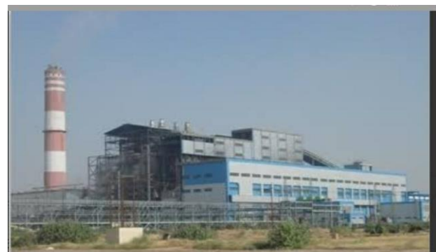
Fig. 4. Barsingsar thermal power station
