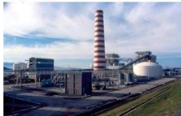
Fig. 2. Surat Garh Super Thermal Power Plant
