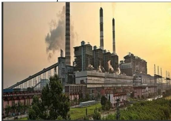
Fig. 5. Chhabra thermal power station
