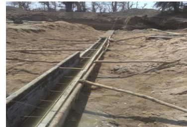
Fig. 2. Casting of reinforcement in curtain wall
