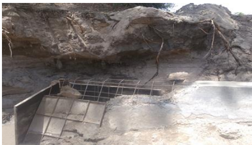
Fig. 1. Casting of reinforcement in cut off wall
