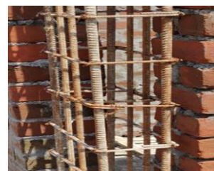
Fig. 5. Joints of ties in alternative position
