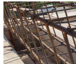
Fig. 4. Joints of stirrups in same symmetry
