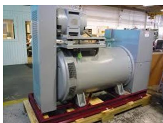
Fig. 2. A typical synchronous condenser
