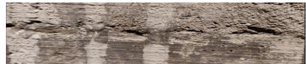
Fig. 3. Collins of concrete in column
