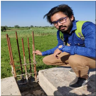
Fig. 5. Placing of interlock system
