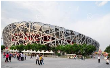
Fig. 4. Beijing National Stadium
