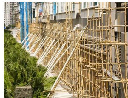
Fig. 7. Bamboo scaffolding
