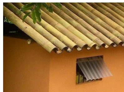
Fig. 8. Bamboo tile roofing
