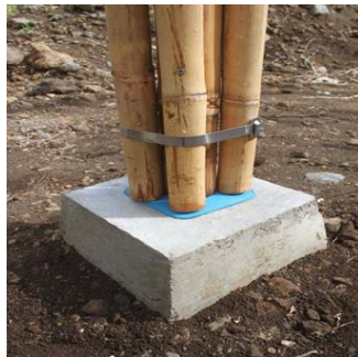
Fig. 4. Bamboo footing
