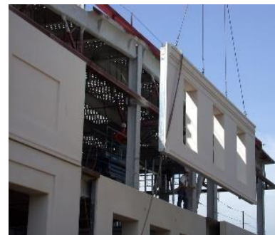
Fig. 3. A building being constructed using prefabricated walls and other elements
