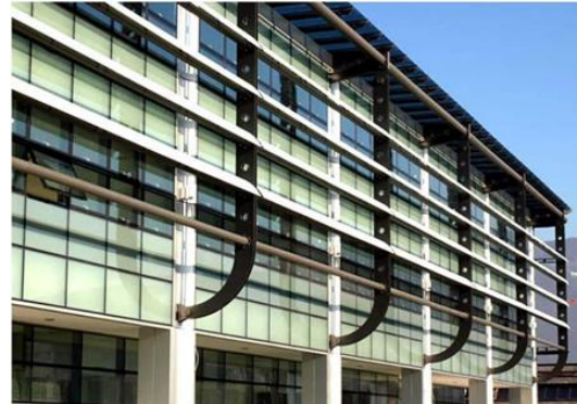
Fig. 4. Brise soleil – shading devices integrated with the building façade
