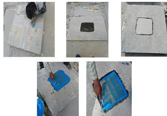
Fig. 2. Application of FRP (CFRP, GFRP, and PPFRP) sheets
