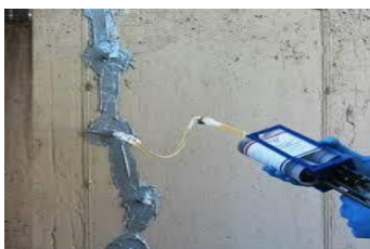
Fig. 4. Epoxy injection to column
