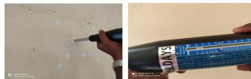
Fig. 1. Rebound Hammer Test
