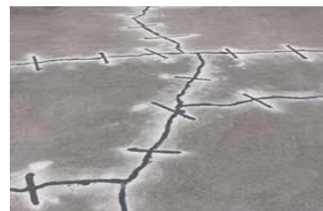
Fig. 6. Stitching of cracks
