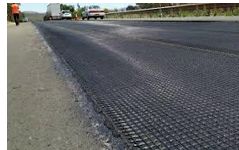
Use of geotextile in road works
