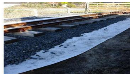
Use of geotextile in railway works
