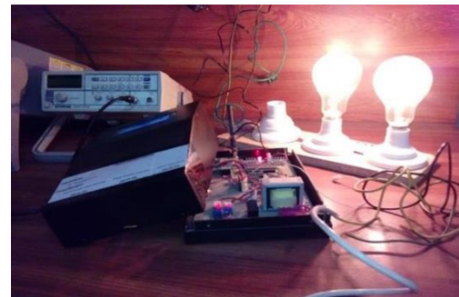
Fig. 5. Smart energy meter in working
