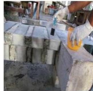
Fig. 4. Application of epoxy and hardener on the beam
