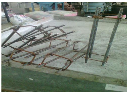
Fig. 2. Typical 12mm high tensile steel reinforcement
