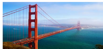
Fig. 1. A typical suspension bridge
