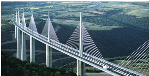
Fig. 2. Cable Stayed bridge
