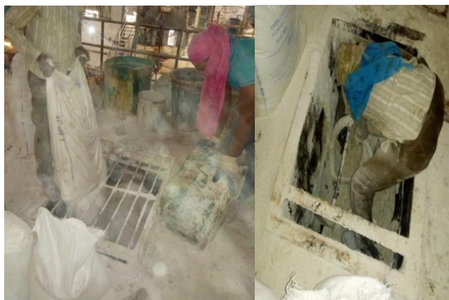
Fig. 4. Pouring raw material and cleaning the mixer
