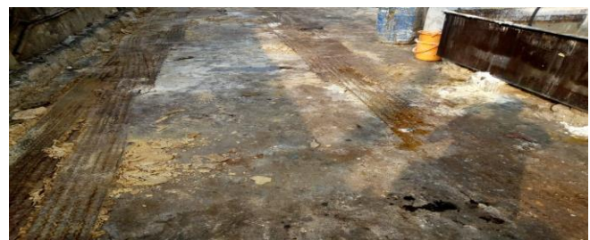
Fig. 3. Bad working condition due to spillage and leakage
