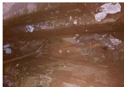
Fig. 7. Blocked drain
