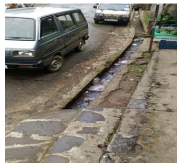
Fig. 6. Drain in the city
