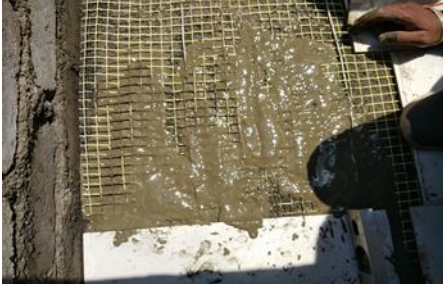
Fig. 1. Making floor heating system
