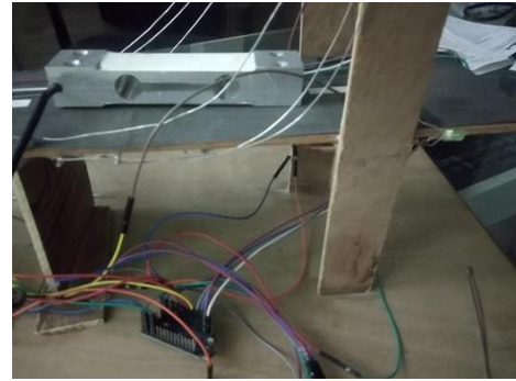
Fig. 4. System deployed on bridge
