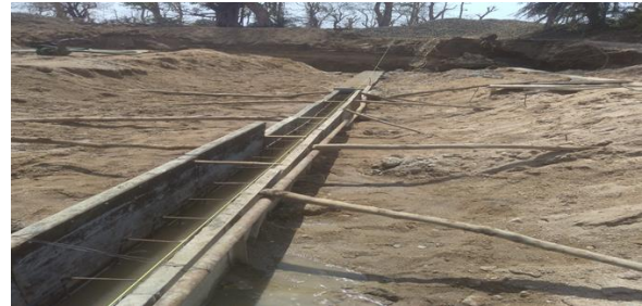
Fig. 2. Casting of Reinforcement in Curtain Wall
