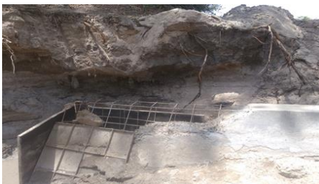
Fig. 1. Casting of Reinforcement in Cut off wall
