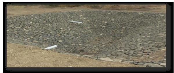
Fig. 12. 3D photo waste water stone stabilization tank [3]
