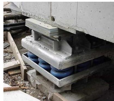
Fig. 4. Base isolation for foundation section
