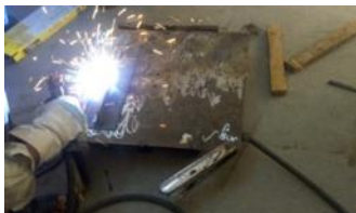
Fig. 2. Preparation of v groove
