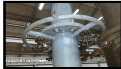
Fig. 5. Grade 1 Pressure tapping
