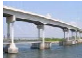
Fig. 1. Sebastian inlet bridge, FL
