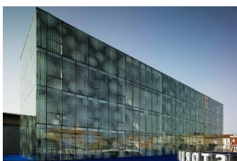
Ceramic printed glass used in facade
