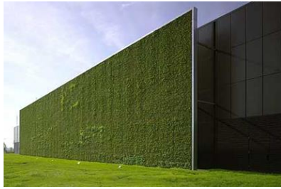
Fig. 4. City Data Center in Frankfurt feature a green wall featuring plants that are irrigated with recycled water
