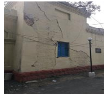
Fig. 3. Deterioration of external rendering
