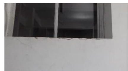
Fig. 11. Horizontal crack
