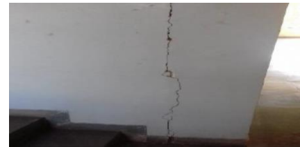
Fig. 10. Vertical crack
