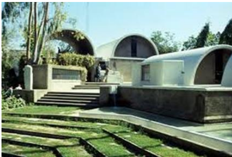
Fig. 5. Exterior view of Sangath
