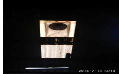
Fig. 7. Turbo ventilator with transparent shed for light ventilation
