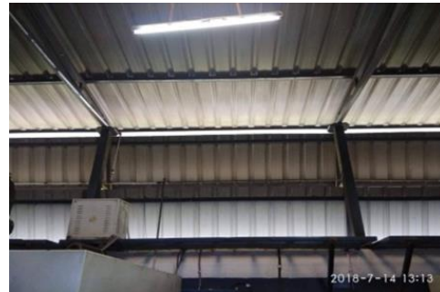
Fig. 8. Alternative shed arranged for cross ventilation
