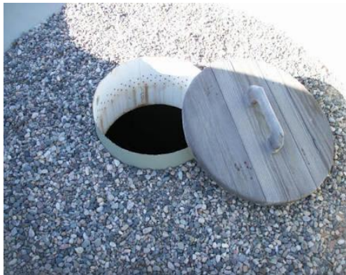
Fig. 5. Cistern with small pores and lid
