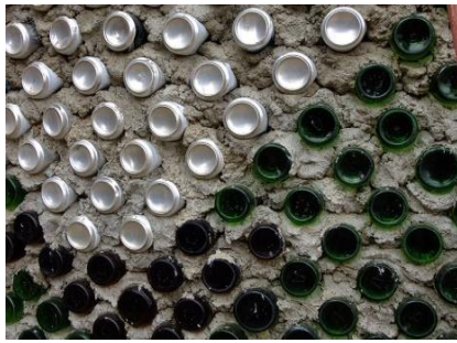
Fig. 10. Waste cans and bottles wall construction
