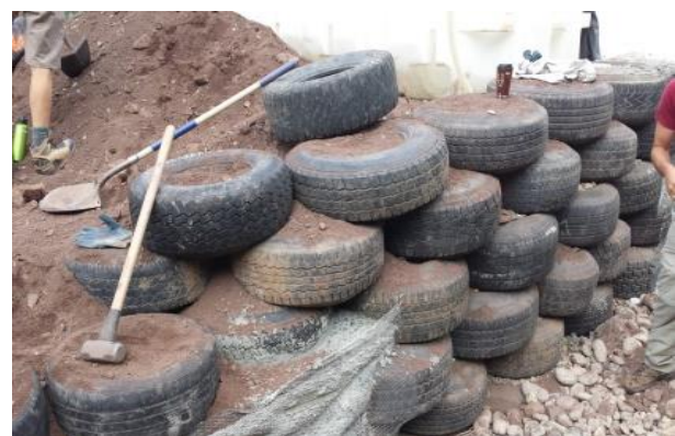
Fig. 8. Tyre wall construction
